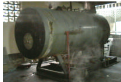
Figura 2. Caldera Hospital San Jorge
